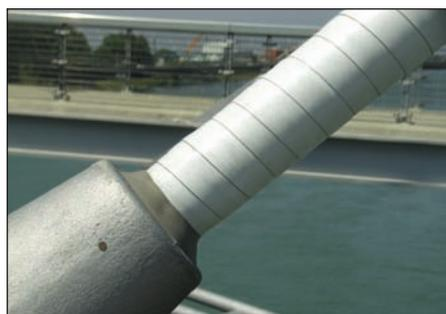
Fig. 7: Sealing at the deck anchorage
