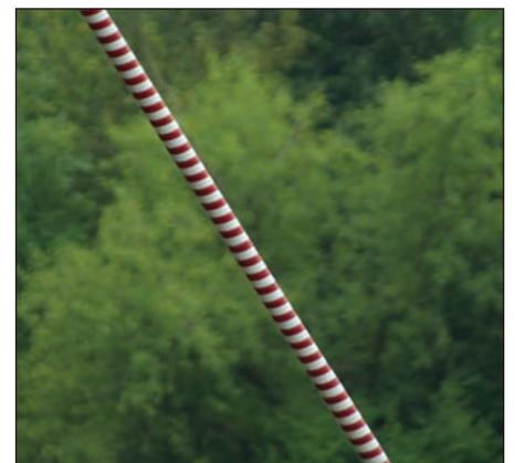
Fig. 10: Wrapping method applied for signal marking
