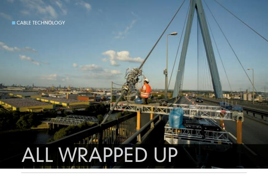
Fully-locked cables on one of Germany's most heavily-used road bridges have been thoroughly inspected and wrapped to protect them from corrosion
