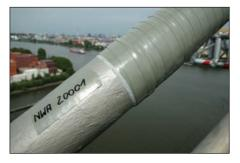
*Fig. 9: Connection of the tapes to the painted rope at the deck anchorage*
