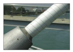
Fig. 7: Sealing at the deck anchorage
