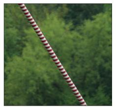
*Fig. 10: Wrapping method applied for signal marking*
